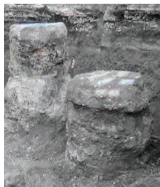
**Figure 4: Photograph of jet-grouted column**
